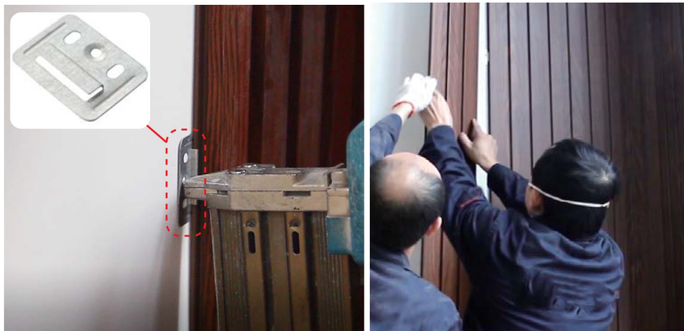
Step3 Fix the wall panels to the wall in turn with clips
