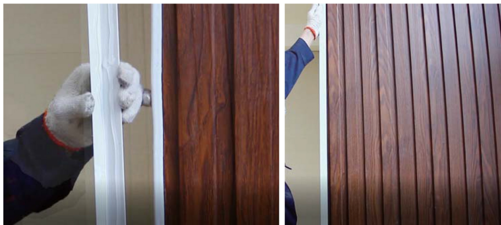
Step4 Glue the L corner and stick on the wall panel, the installation is finished
